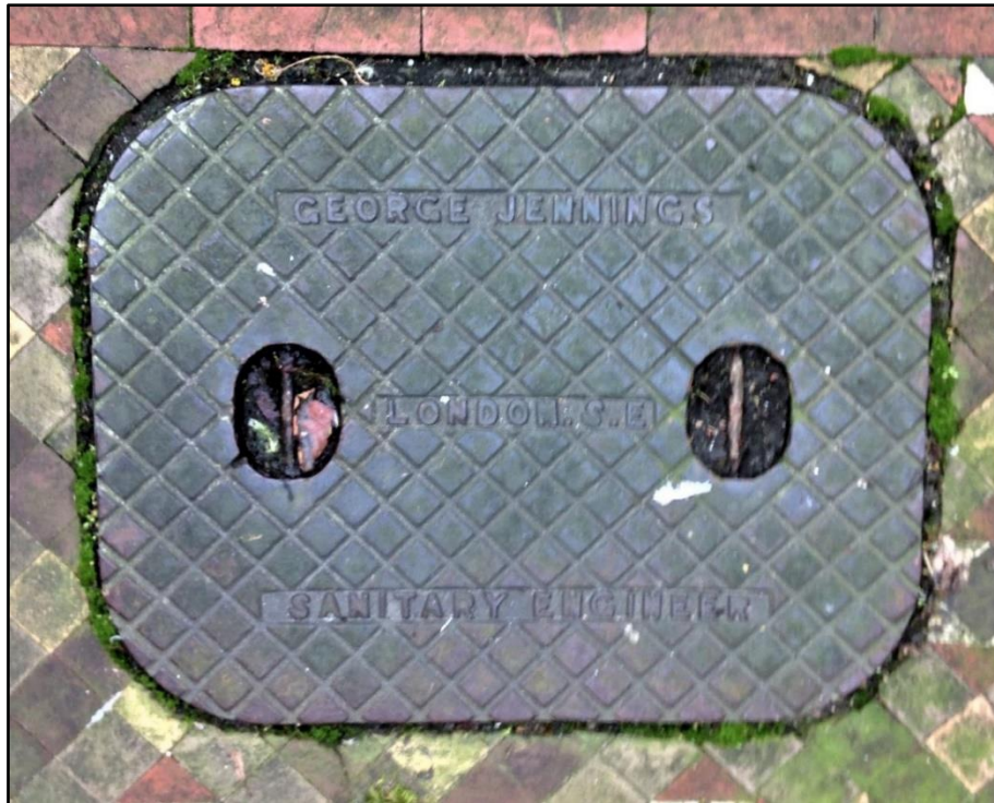
Drain cover in Canute Road, Southampton
