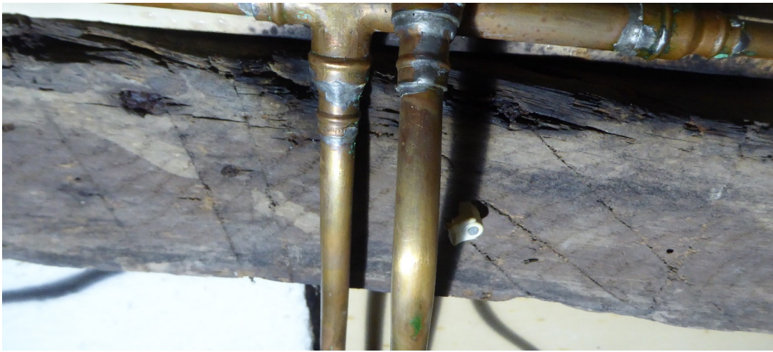
45 Bugle Street. Beam 7. Carpenters' assembly marks
