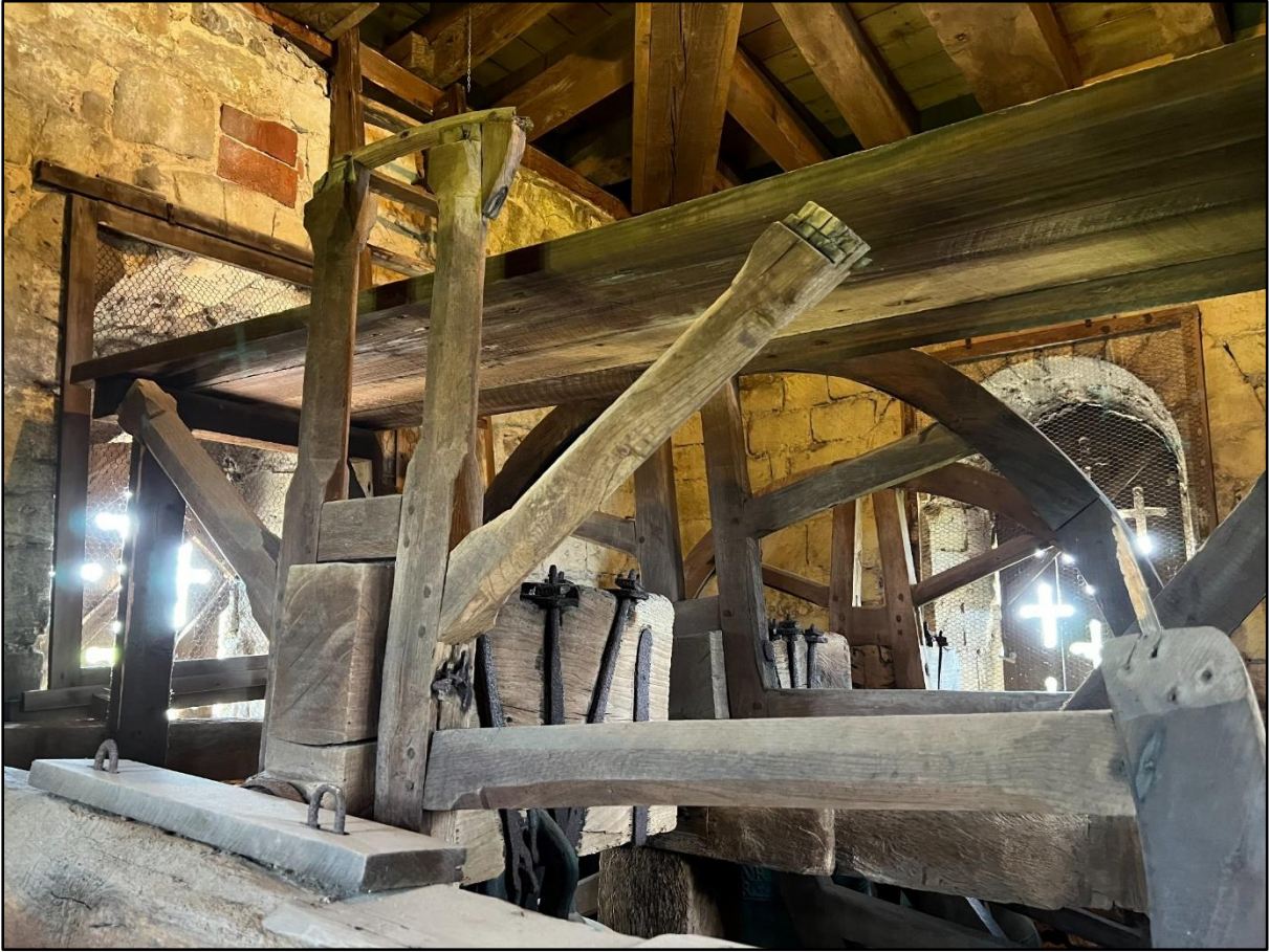
The Bell Headstocks hold the bells in place and allow them to be turned when rung.
