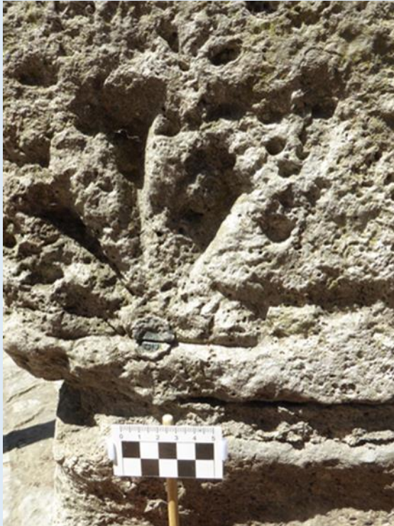
Above: Inverted cut benchmark with bolt head. Right: Enlarged image of bolt head (see text). Photos – K Wardley
