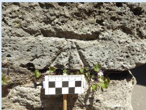
Above: Arrow incised on lintel stone above eastern doorway. Left: OS benchmark cut into cornerstone. Photos - K. Wardley
