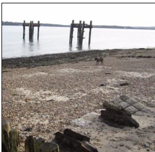
Dolphin mooring posts at Lepe, with remains of concrete beach hardening mats (centre right) and winch bases. Photo: S Hanna
