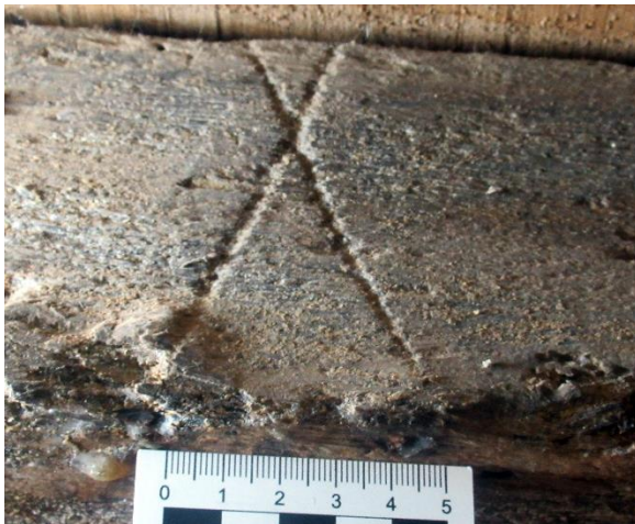
Fig 9 Shop. X-shaped carpenter's assembly mark on ceiling joist
