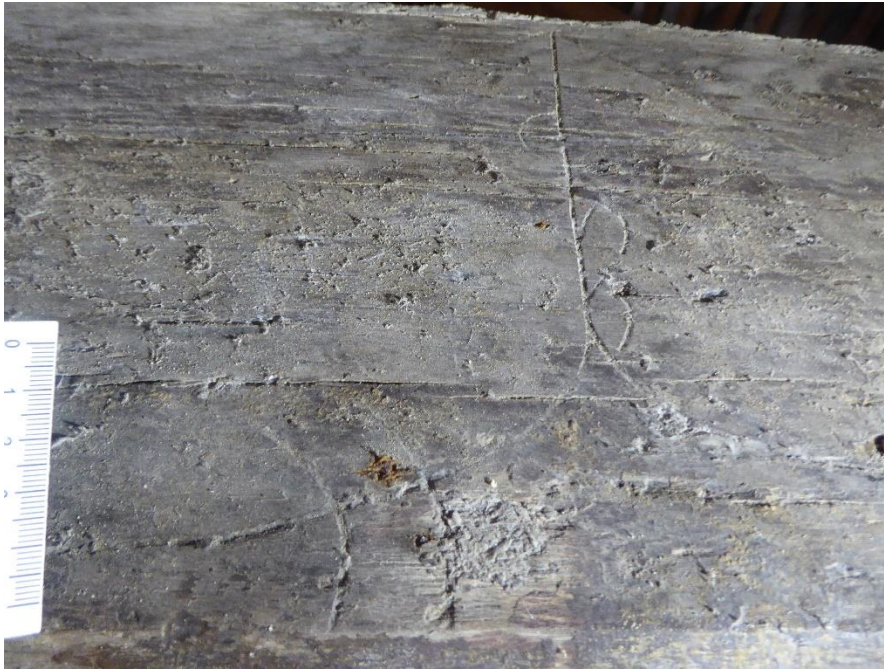
Fig 12 Front bedchamber. Truss B. Merchant mark, base with extended arm
