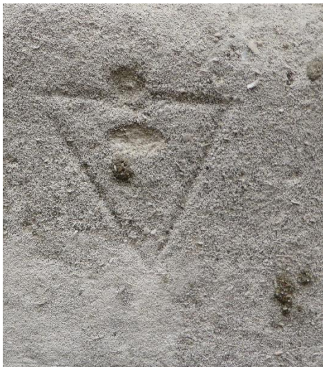
Fig 1 Exterior south wall. Mason's mark
