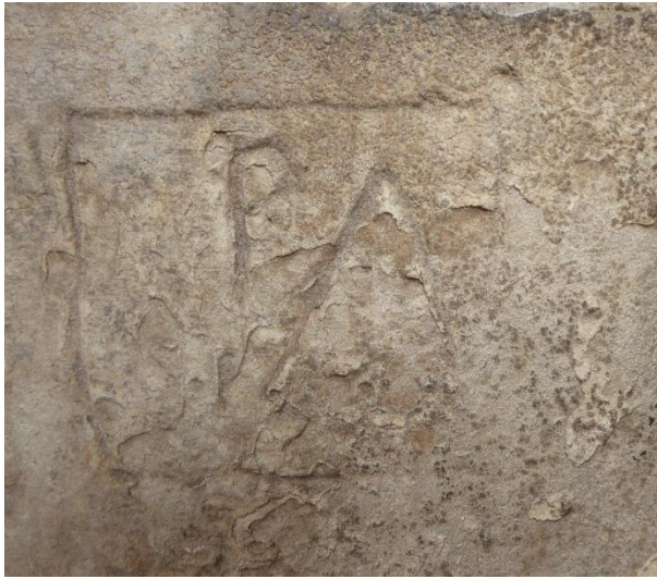
Fig 2 East wall, south side of doorway. Boxed initials PA
