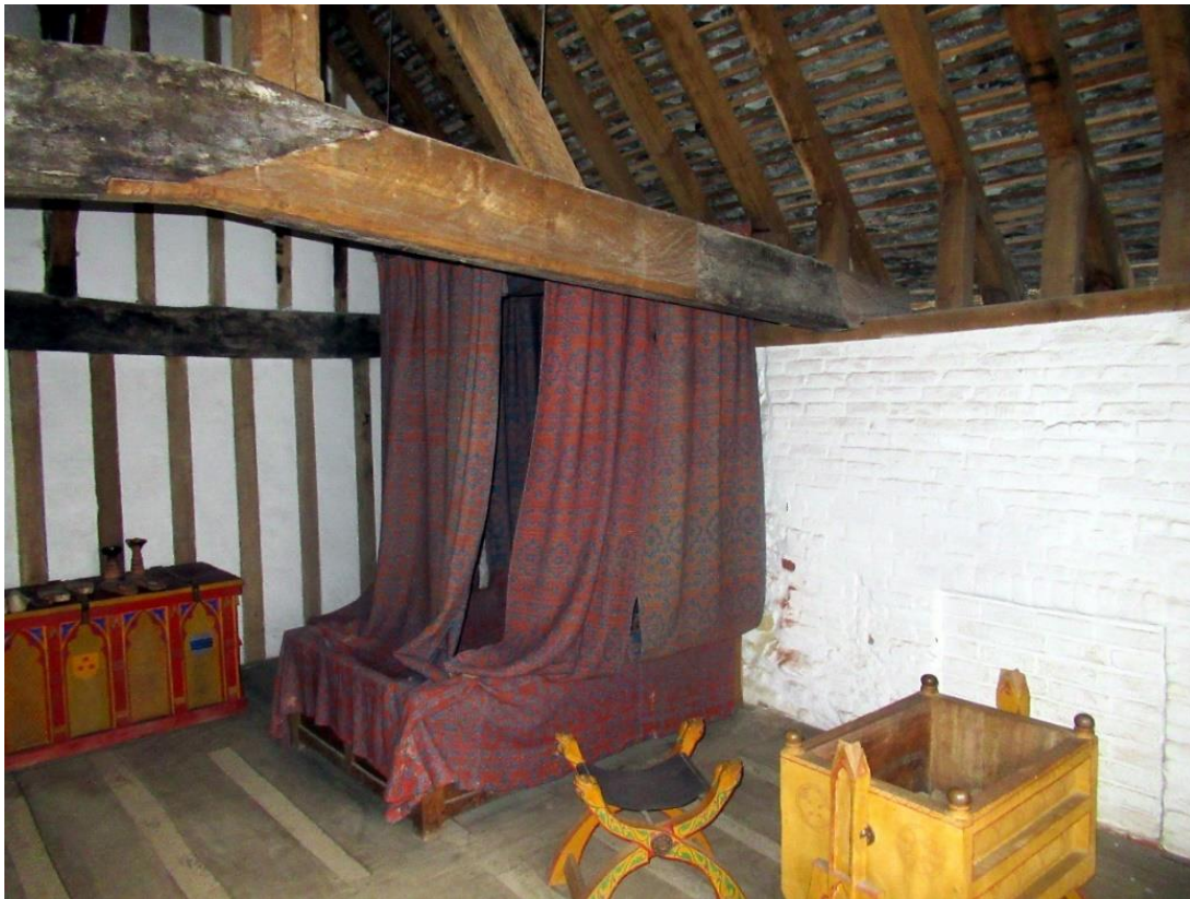
Fig 14. Bedchamber, tie beam, Truss C
