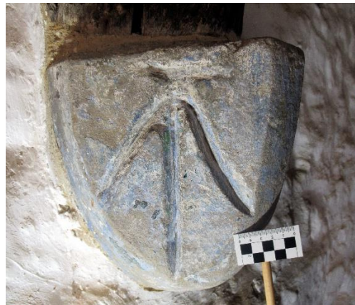
Fig 6 Inner room, south corbel, arrow
