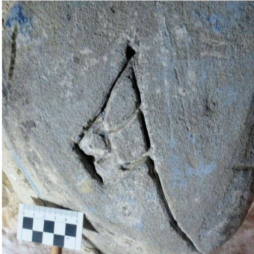
Fig 5 Inner room, south corbel, flag shape
