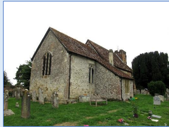
Figure 2 St John's from the NE
