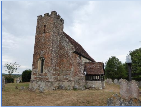
Figure 1 St John's from the SW
