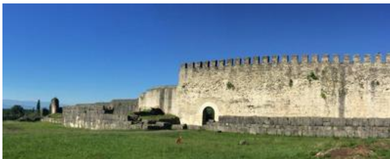
View of walls showing variation in construction methods. Photo: P.Everill
