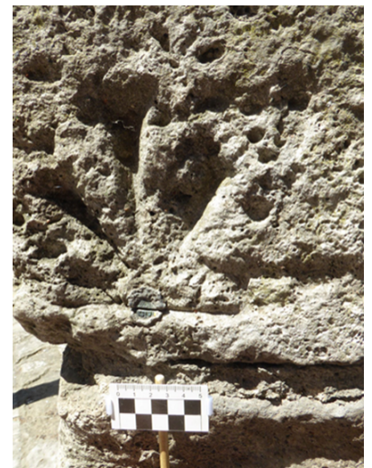
Left: OS benchmark cut into cornerstone. Photos - K. Wardley
