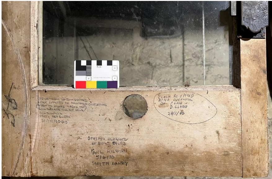
18 Tower. Turret clock case door with pencilled repair records
