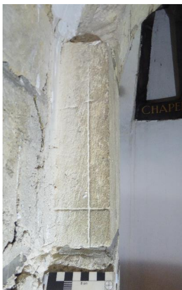
19 Nave, south side. Masons’ marking-out lines on archway
