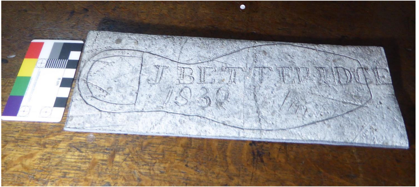
17 Lead sheeting from tower roof. Shoe sole, J. Betteridge 1830
