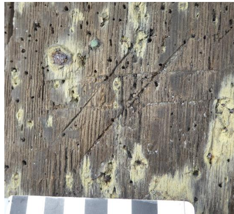
9 North door. “Hache “ shape
