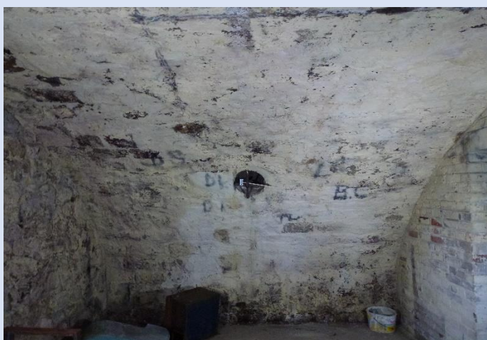
Fig. 2 Black painted letters on north wall of furthest vault
