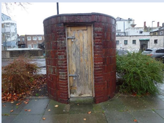
Fig. 1 Cylindrical brick built entrance to the vault via a concrete spiral staircase
