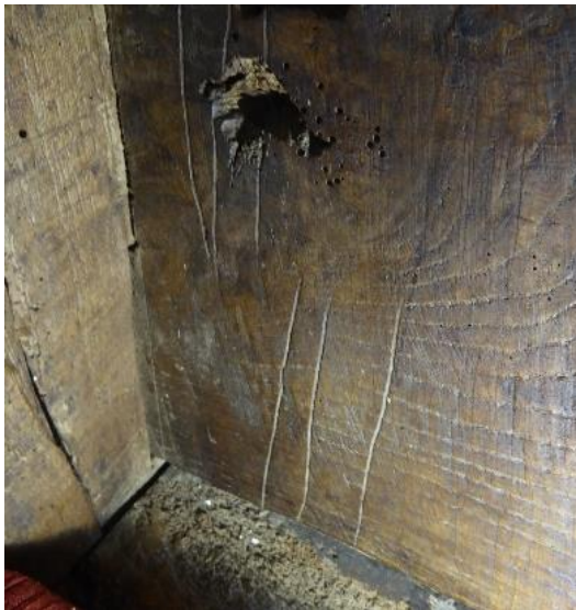
24 Pew back, possible carpenter marks, 2 sets of 3 lines
