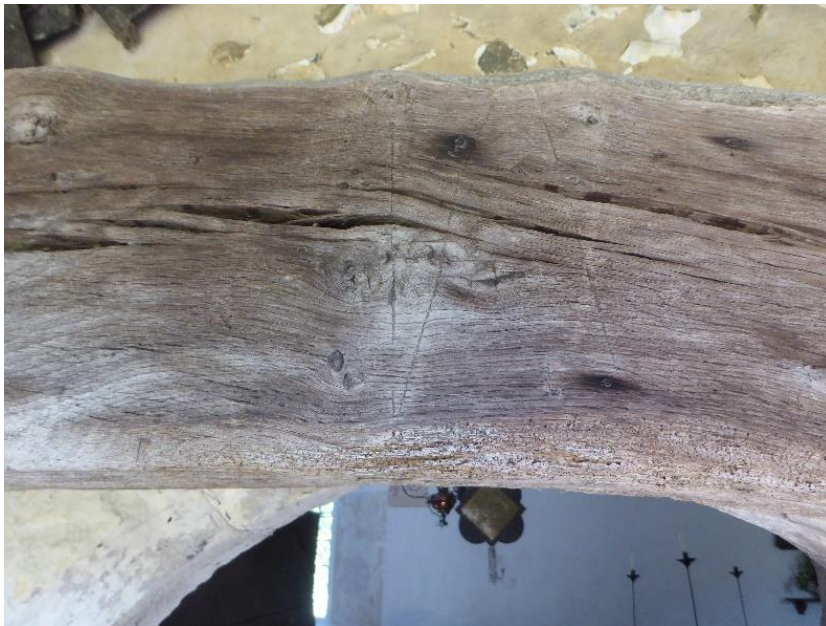
7 Carpenter mark, possibly VI, on tie beam, porch
