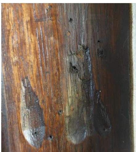
21 Burn marks on west face of rood screen
