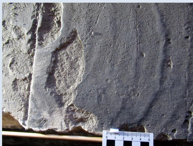
Fig. 5 – Incised “GB IM 1971” and vertical line on the sill of the central window
