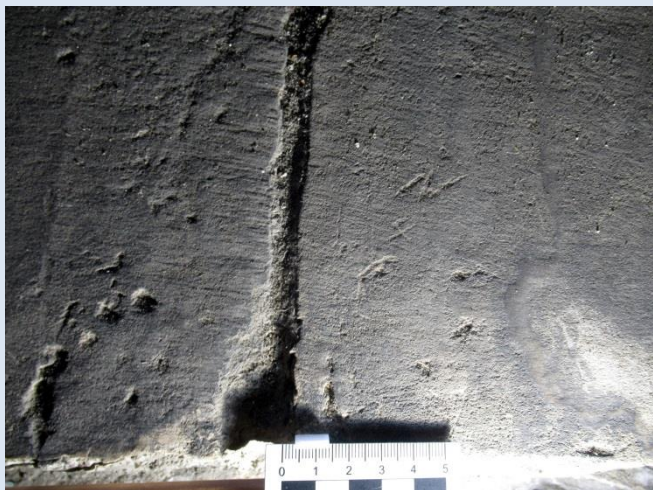
Fig. 4 – Incised “N4C” on the sill of the central window
