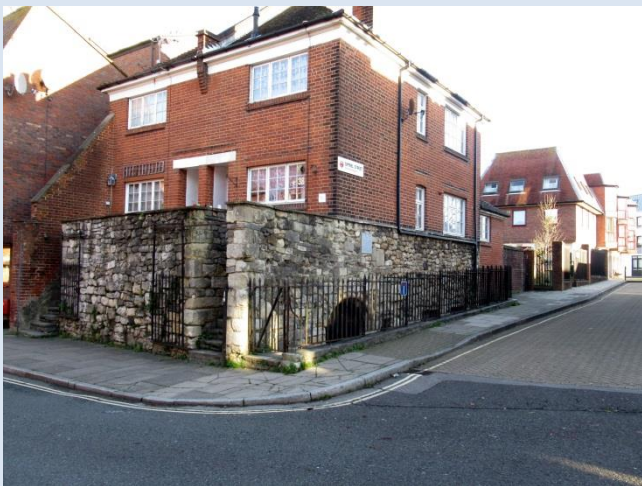
Fig. 1 – Access to the Undercroft
