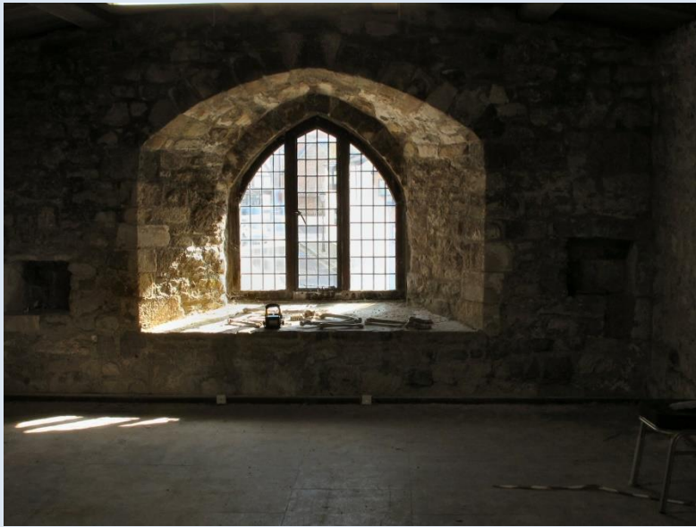
Second floor East window showing aumbries either side of window
