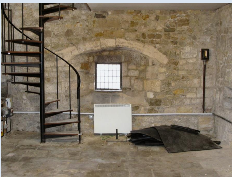
A View of the first floor looking west. A modern spiral staircase leading up to the second floor is located in the Southwest corner
