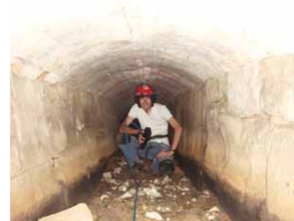
A disused conduit for the Lockburn
