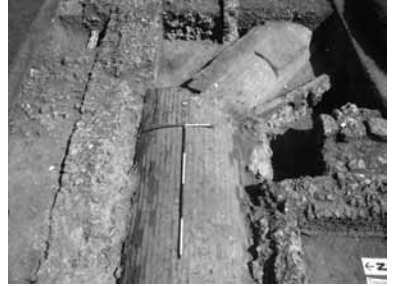
A culvert carrying the lockburn at the rear of the demolished south range. Photo: Chris Sellen
