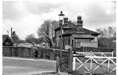
The old level Crossing in Bishops Waltham © Ben Brooksbank
