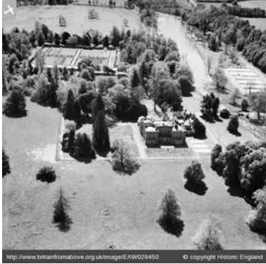
Warnford House/Belmont just before demolition
